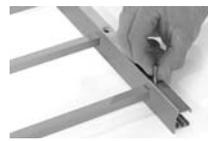
**Step 8.** Position all Phillips head aluminum picket hardware kit screws in bottom rails.
