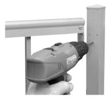
**Step 4.** To secure the end bracket to the post use (3) #8 x 1/2" stainless steel self-tapping screws (furnished) for each end bracket. Follow same procedure for the remaining three rail section ends. **Installation Tip:** Note that a 6" shaft extension fitted to the phillips screwdriver bit aids in the job and helps to prevent scratching the paint.
