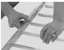
**Step 7.** After the last picket is in place, insert and hand tighten the end picket screw to keep assembly together.
