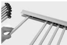
**Step 4.** Center each picket to pencil mark on top rail. **Do Not** tighten stainless steel screws at this time.
