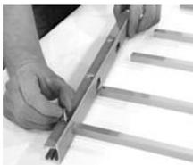
**Step 6.** With end picket screw in place, ease the next picket in square hole (gradually one at a time) until all pickets are in place.
