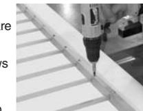
**Step 10.** With a battery operated adjustable clutch drill, turn stainless steel screw so point of screw bears against flat inside surface of top rail. The reason for this is to hold the picket in place at the pencil marked line on the top rail. Set the drill clutch at a low torque setting and low speed to prevent over tightening of component parts.
