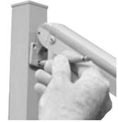
**Step 2.** Drill 1/8" holes in post for mounting location of top and bottom rails.
