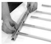
**Step 6.** With end picket screw in place, ease the next picket in rectangular slot (gradually one at a time) until all pickets are in place.
