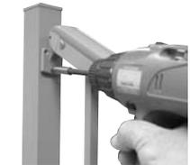
**Step 4.** Position assembled posts and railing onto final mounting location. Use the 2 post base holes as a template and mark mounting holes on platform or floor surface. **Note that the centerline of the post must be a minimum of 3-1/2" from outer edges of concrete platform.**
