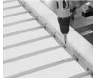
**Step 9.** With all picket screws in place, tighten all screws. **Do Not** over-tighten. Start with lowest clutch torque setting, then gradually increase for proper torque.
