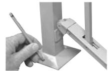
**Step 5.** The hole to be drilled into the mounting platform should be angled, so it is approximately perpendicular to, (or 90 degrees to) the angled, sloped post base. The diameter of the fastener used must be a minimum of 5/16". The exposed fastener and washer should be stainless steel. Two drilled holes (one on opposite sides) are required for each post. **CHECK APPLICABLE STATE, LOCAL, AND FEDERAL BUILDING CODES FOR SPECIFIC REQUIREMENTS FOR POST BASE MOUNTING.**
