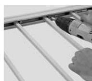
**Step 10.** With a battery operated adjustable clutch drill, turn stainless steel screw so point of screw bears against flat inside surface of top rail. The reason for this is to hold the picket in place at the pencil marked line on the top rail. Set the drill clutch at a low torque setting then gradually increase for proper torque to prevent over tightening of component parts.
