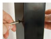
Feed the tension stud through the end post to meet the receiver. By hand, screw the receiver onto the tension stud at least 6 full turns.
