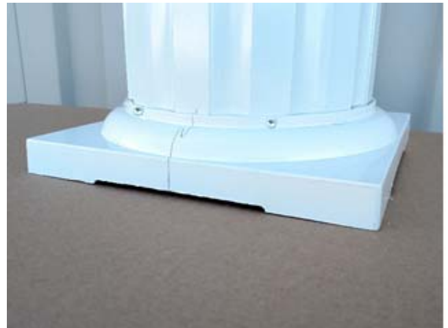
Photo 2: After cap/base installed against column
